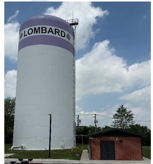
North Ave Standpipe and Pressure Adjusting Station Rehabilitated 2024
