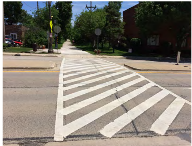
The intersection of Main Street and the Illinois Prairie Path was retrofitted with a pedestrian refuge island, yet the four travel lanes may intimidate trail users.
