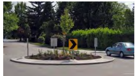
Level 4: Traffic Calming
