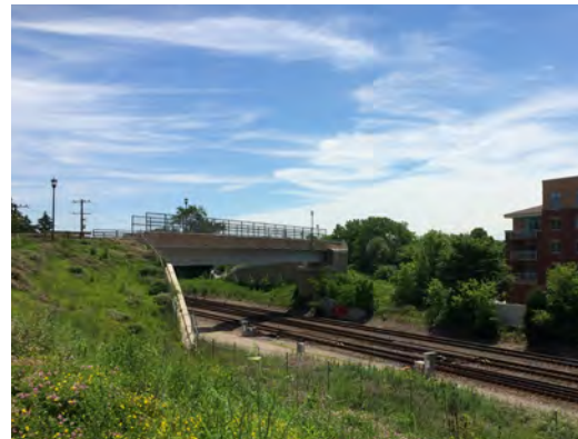
Great Western Trail Overpass at Metra Train Tracks near St. Charles Road
