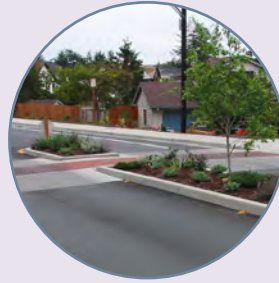
Median Refuge Island
