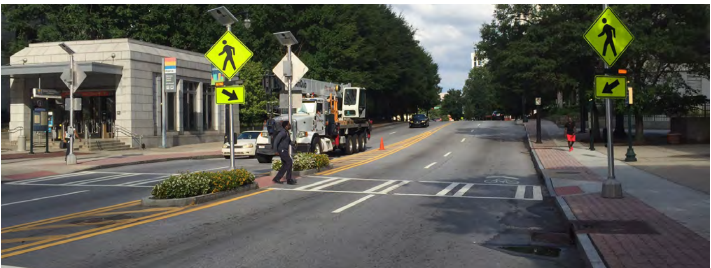
An example of a Rectangular Rapid Flash Beacon (RRFB) and pedestrian refuge island.
