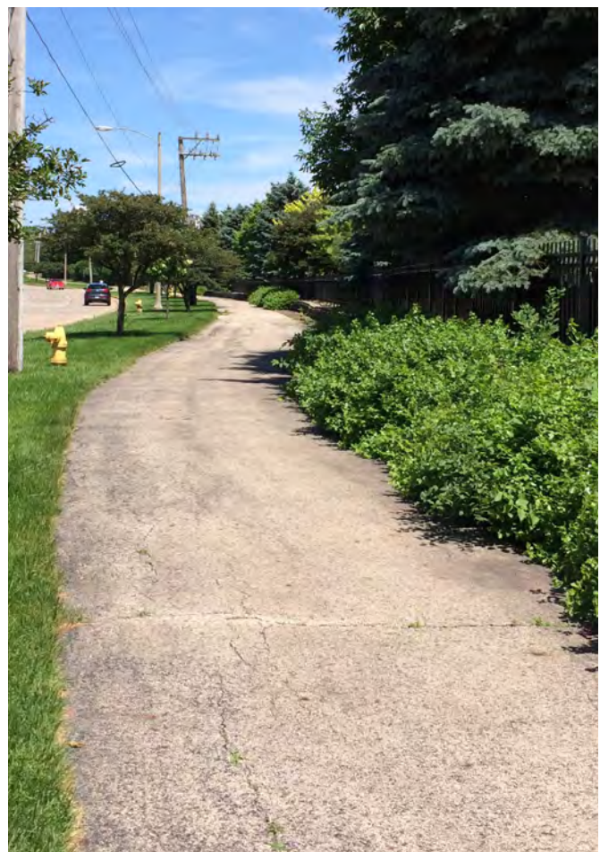
22nd Street and Finley Road sidepath
