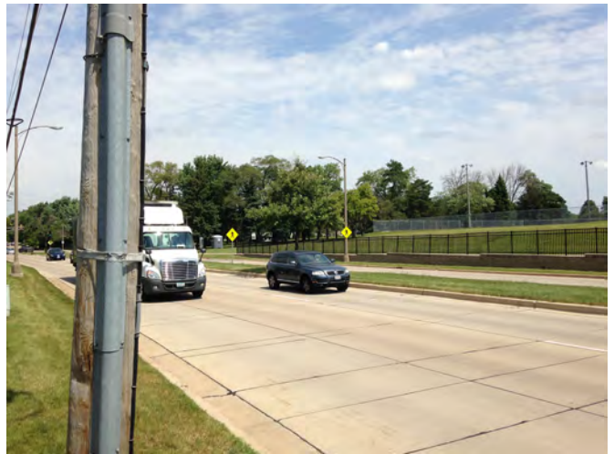
In contrast to the photo above, residents reported difficulty bicycling and walking along busy, car-oriented roadways.
