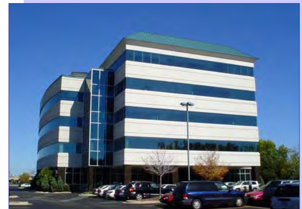
Heron Point (below) was completed in 2002 and features 98,604 sq. ft. of Class A office space as well as an on-site, 114-room Fairfield Inn & Suites hotel. Acosta and Staples are major tenants.
