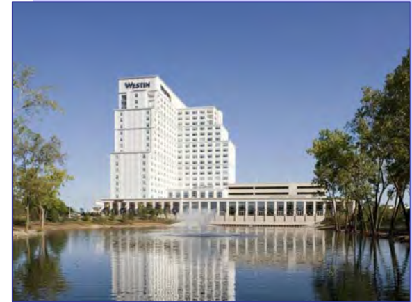
The Westin Lombard hotel conference center (above) is a 440,000-square foot, 18-story building with 500 hotel rooms and suites, 55,500 square feet of meeting space, and amenities commensurate with a full-service, convention-oriented five-star hotel.
